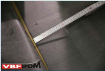
15. Overlap van 10 cm tussen VBF-EPDM membranen.
