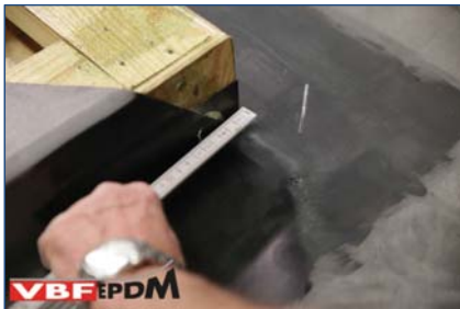
64. Opmeten Detailfolie minimaal 10 cm overlap.
