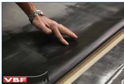
7. Controle droging Singleply Primer.
