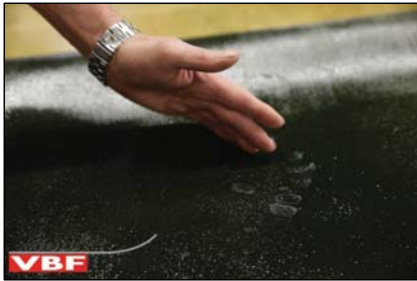
12. Contactlijm is handdroog.
