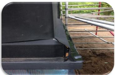
Virtually seamless VB-EPDM facade cladding can be supplied in any shape or size. This reduces the number of necessary seam joints at the construction site and therefore saves valuable application time. VB-EPDM sheeting is UV resistant and elastic. This makes the material ideally suited for use with expansion joints, where heavy demands are made in respect of permanently sealing building components that move in relation to one another.
